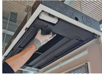
▶ Remove the condensate tray.
